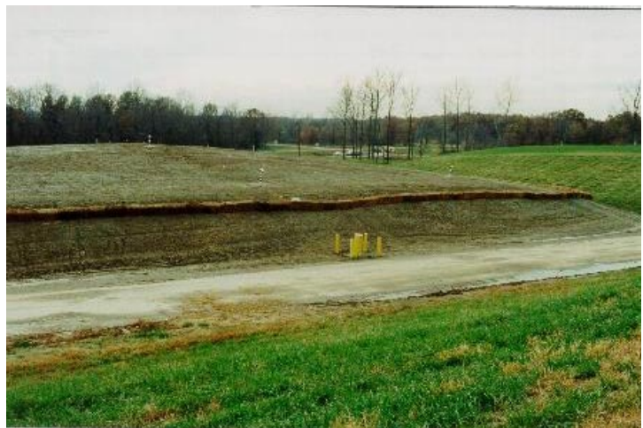
Existing landfills have been capped, monitoring wells have been put in place, and controls have been installed to limit erosion of sediments and spread of contamination.
