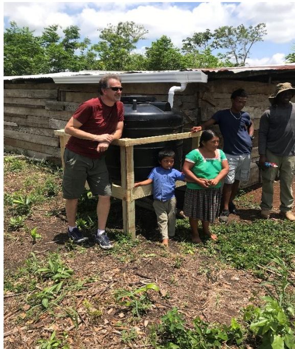
(One of the final water tanks we installed)
