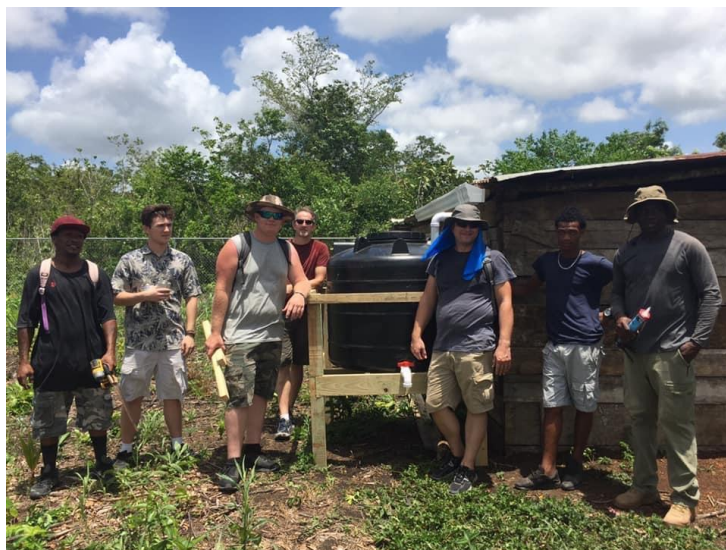
(Some of the team and I with one of the water tanks we installed)
